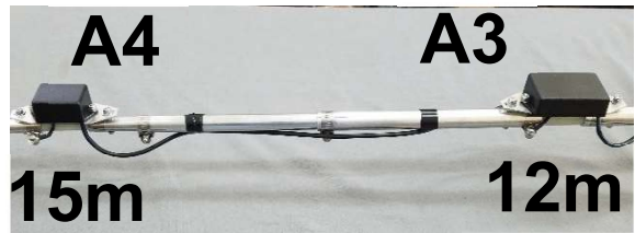
FIGURE 91 Final taped cable under sections A3 and A4 from 15m to 12m module.
